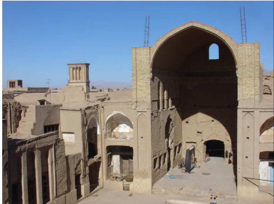
Fig. 7. Changing the frame of the entrance of tanabi space from vertical frame to horizontal frame in Hossinnyan's house, Yazd (Archives of the General Administration of Cultural Heritage of Yazd).
