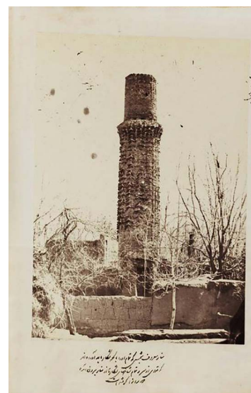
▲ Fig. 8. The oldest photograph of Shams-e -Tabrizi minaret, which was taken by Ali Khan Vali in 1297 AH. Photo caption: “The famous Shams-e Tabrizi minaret is built with animal heads. A small proportion of the heads and entire horns are embedded outside the minaret, engulfing the building” (Credit: Harvard University; iif.lib.harvard.edu/manifests/view/drs:6665026$50i ).
