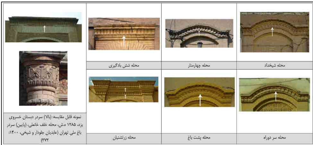
Fig. 6: Use of molded brick in the facade of houses (author, 2023).
