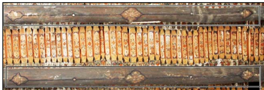
Fig. 34: A Toranj with connected Toranj heads in the Zarir Mosque (Authors, 2019).
