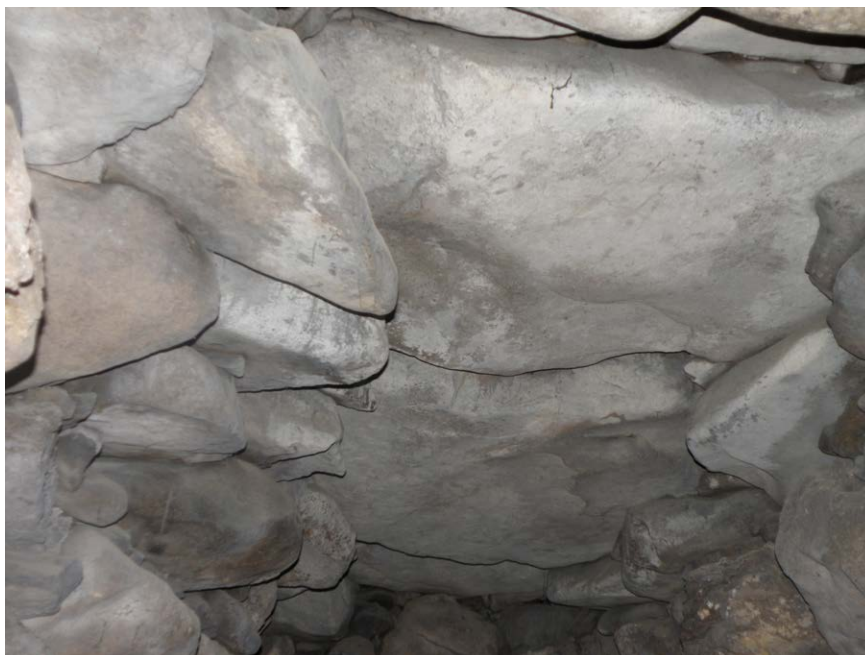
◀ Fig. 5: Large stone slabs covering the tomb's roof, viewed from the interior (Authors, 2024).
